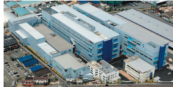
Hisaka Works, Ltd. Konoike Plant (Osaka, Japan)
