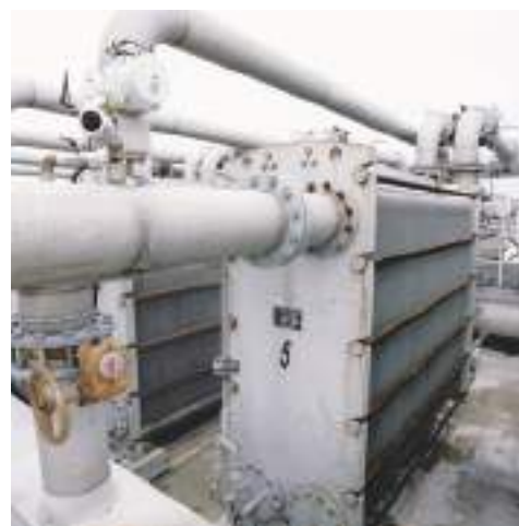
Heat exchange of black liquor / white water, oven blow gas condensation, waste heat recovery
