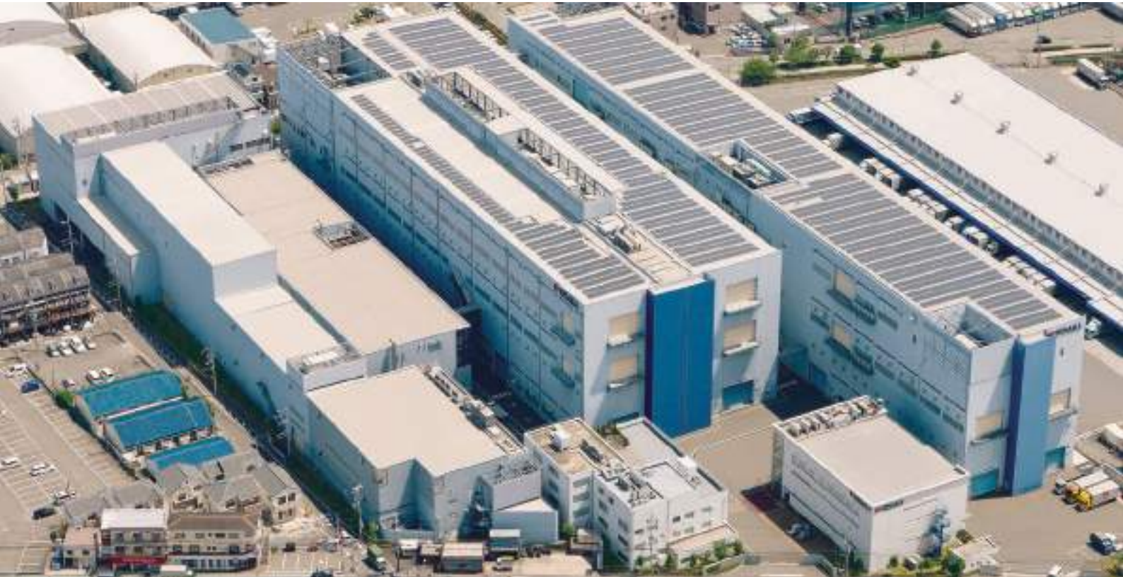
HISAKA WORKS / Konoike Plant
